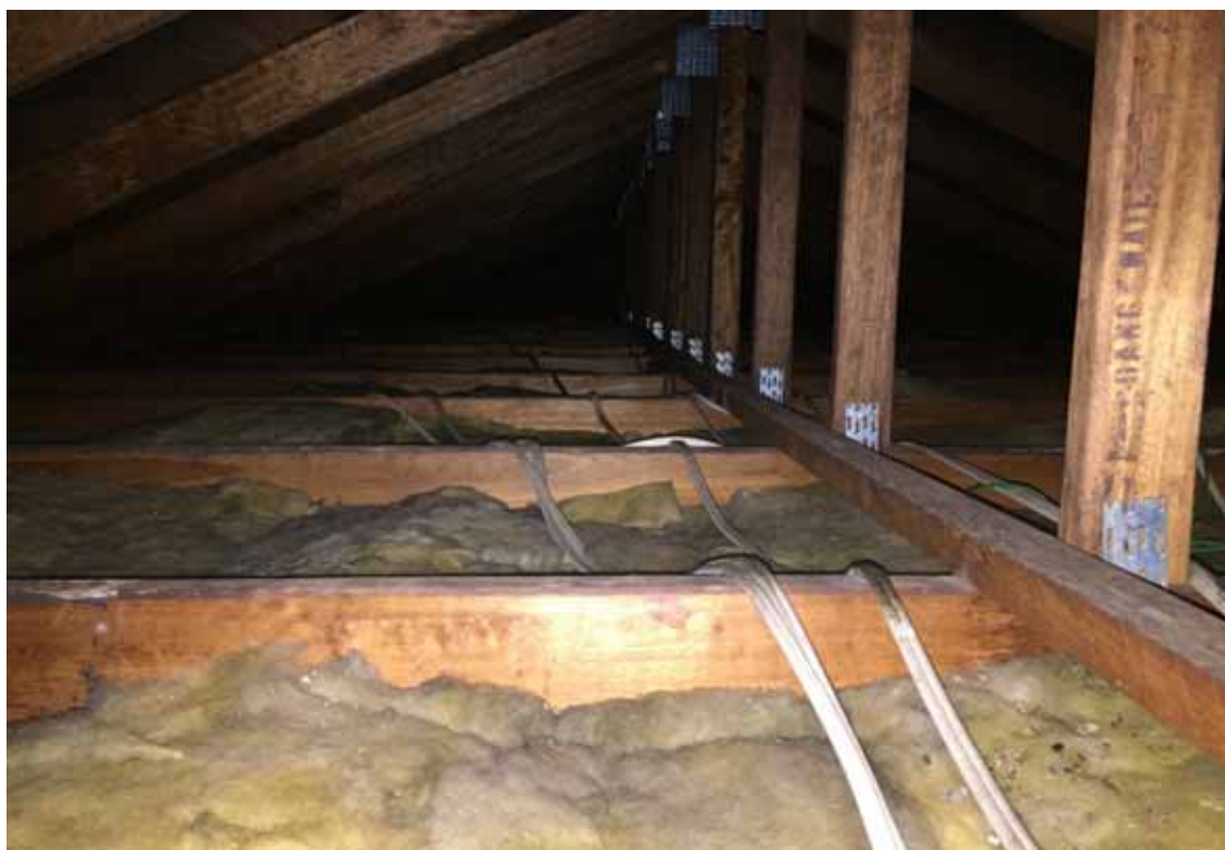
Photograph 22: Unit 3, ceiling cavity, settled dust (lead) and insulation batts (SMF).
