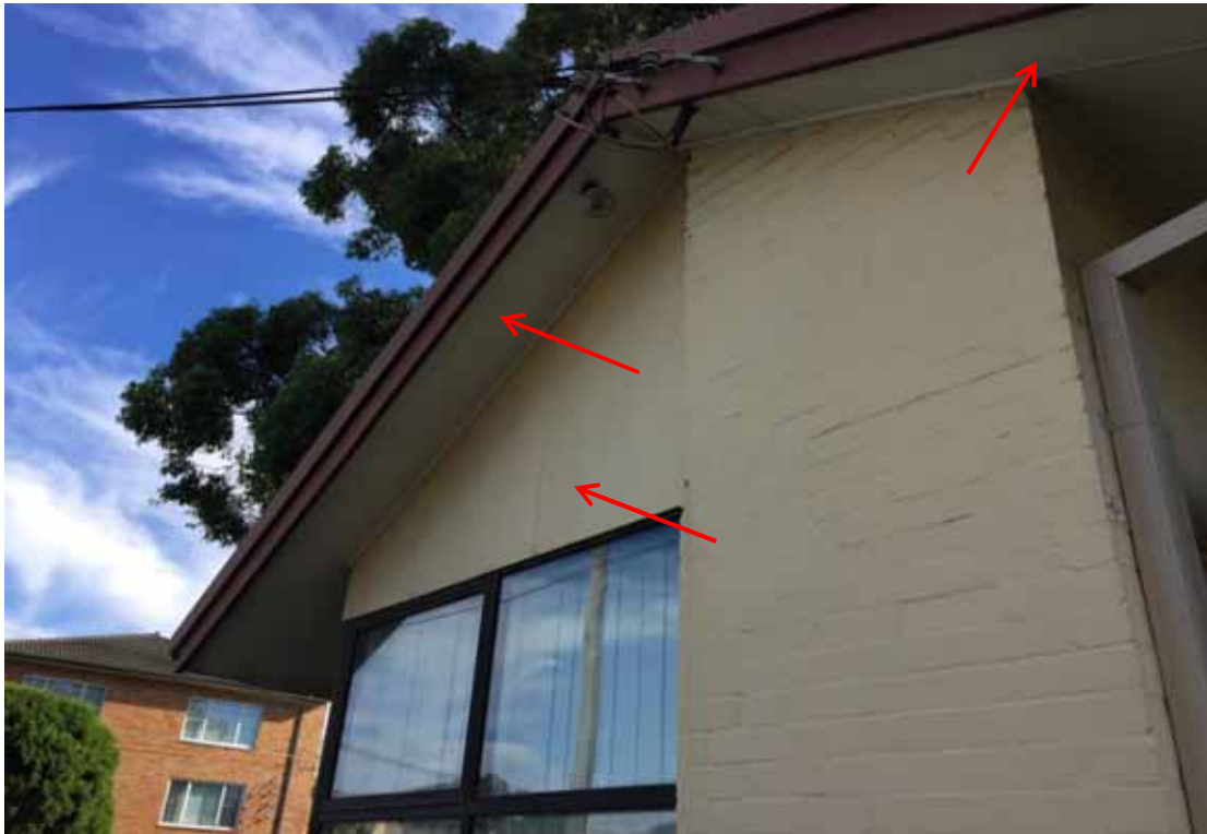
Photograph 16: Unit 3, eaves and gable lining, fibre cement sheeting (asbestos).
