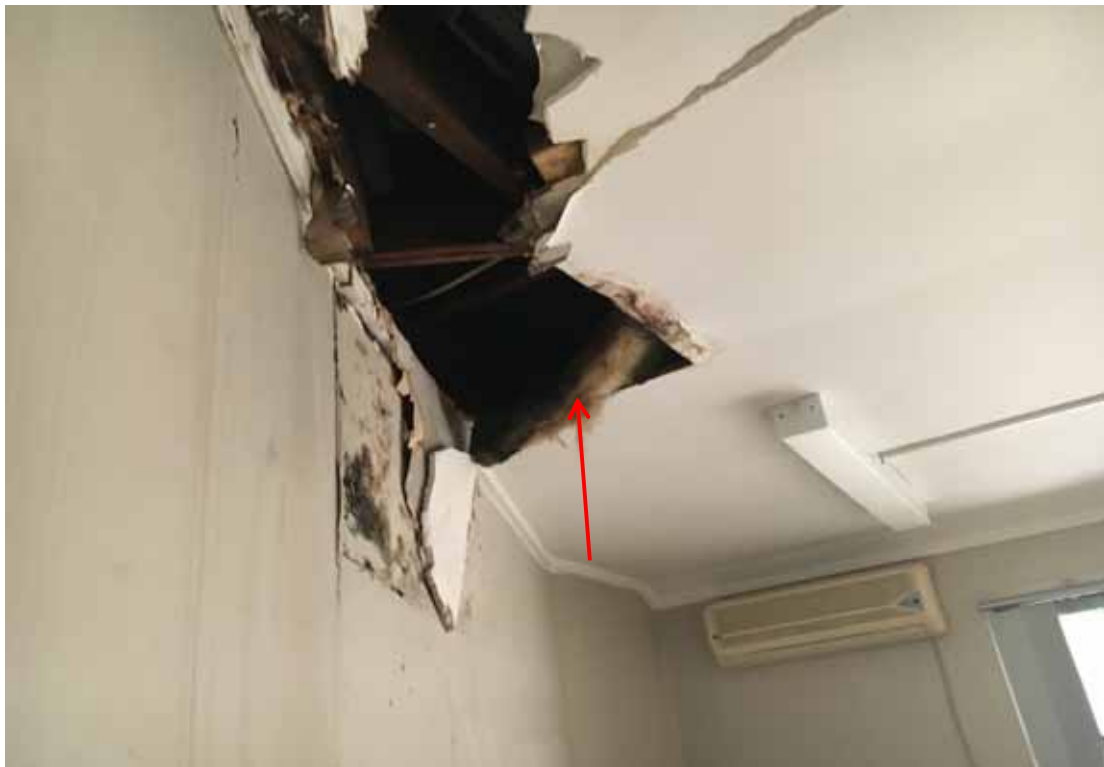
Photograph 6: Building 1, internal, ceiling space throughout, ceiling insulation (SMF).
